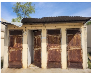
BMW storage area
